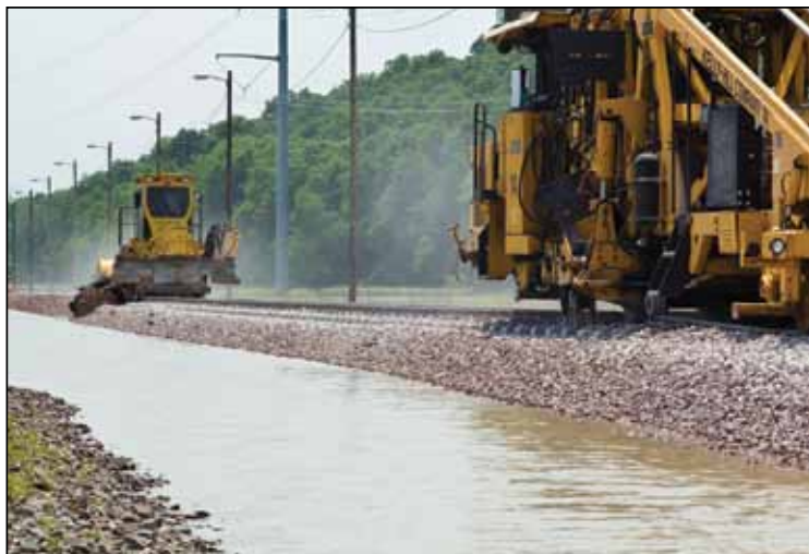
A tamper vehicle uses its "claws" to grab and lift a section of rail/ties, while using vibrating "paddles" to compact the new ballast under the track, effectively raising the rails.
