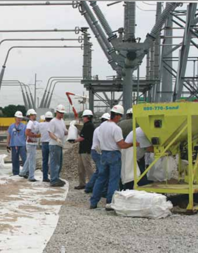
Workers formed an assembly line to build a sandbag barrier to protect the substation at FCS.
