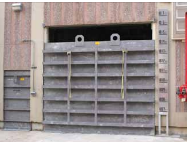
These floodgates were installed on the FCS Intake Structure in early June.
